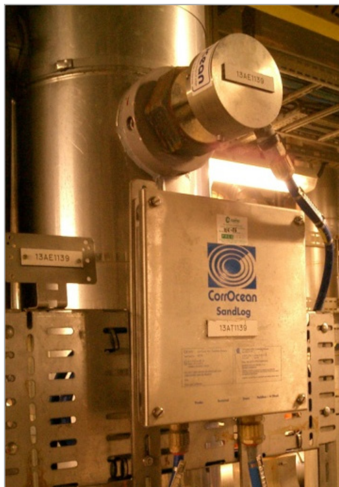
Hydraulic access fitting with Sandprobe and SandLog instrument installed in vertical pipe.
